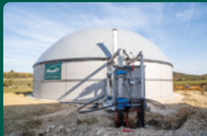
7. Day Pipeline construction completed and ready for operation
