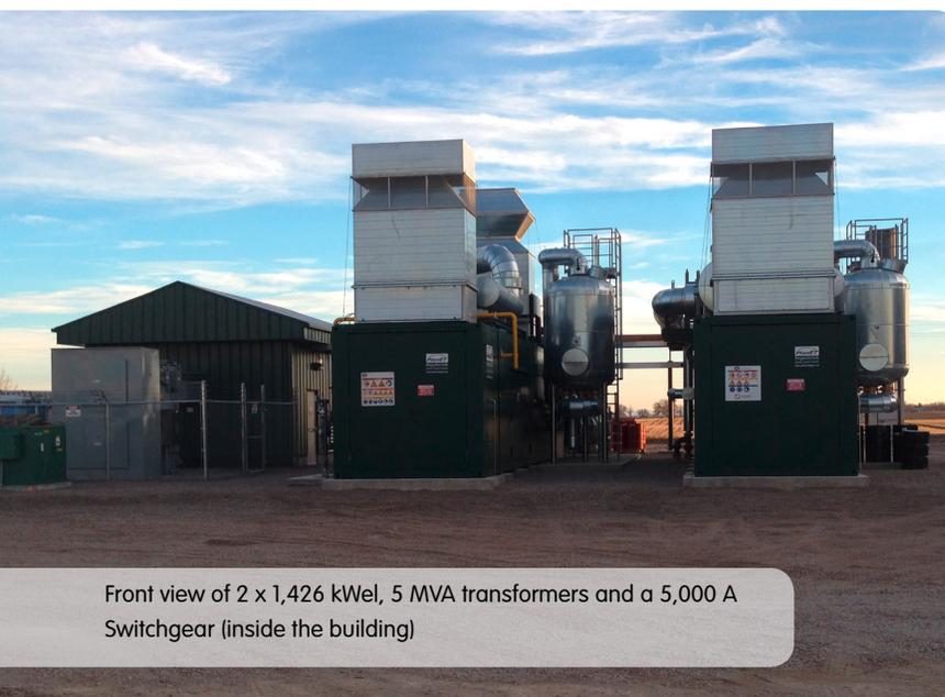
Front view of 2 x 1,426 kWel, 5 MVA transformers and a 5,000 A Switchgear (inside the building)
