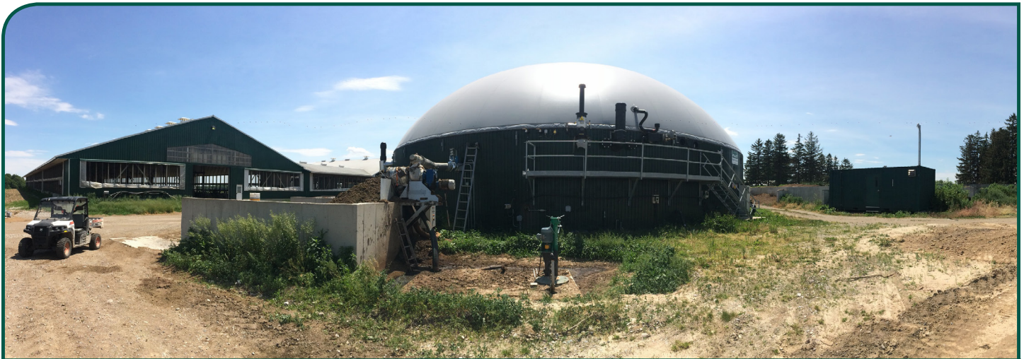
Electrical output: 500 kW | Commissioning: 2013 | Cofermentation AD plant
